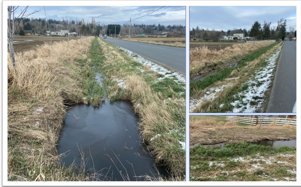
Drainage on Martindale Flats
